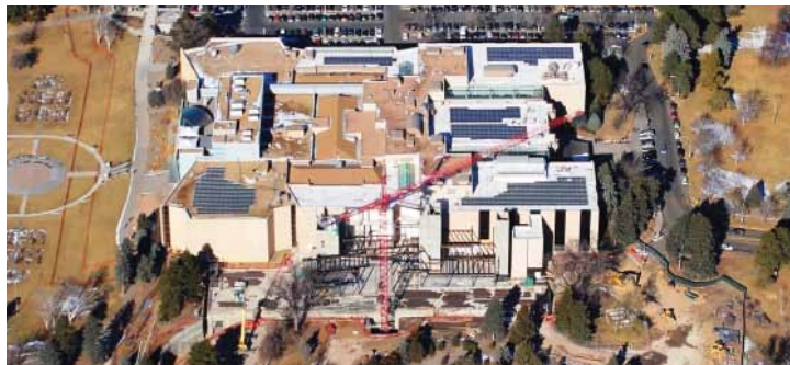
By this point in early 2013, the two underground storage collection levels had been constructed on the site, ready for erection of the steel to support three upper floors.
