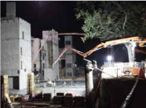
A fall 2012 concrete pour before sunrise delivered 1,000 cubic yards of concrete pour at one time -- about 7% of the total amount used during the project's construction.
