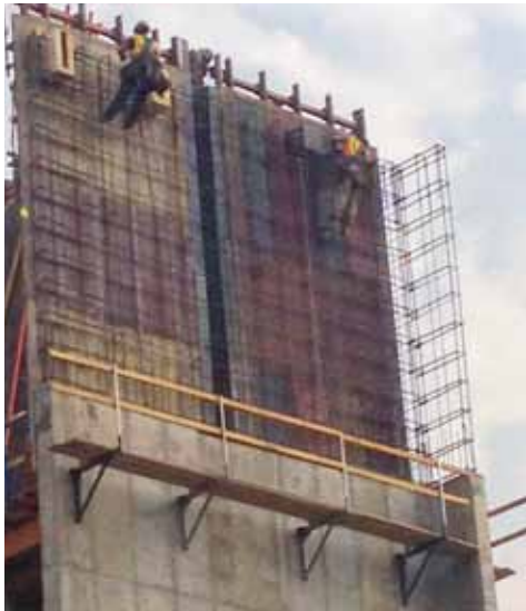
The concrete and rebar "walls" seen under construction were an initial component of the project.
