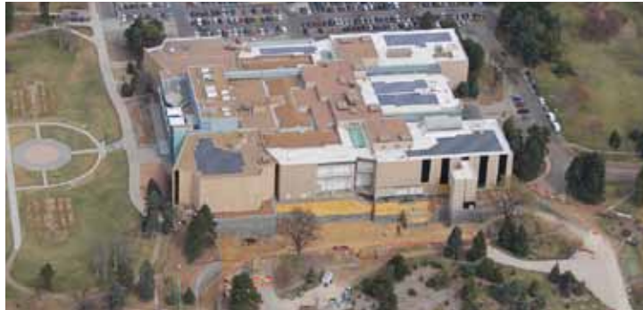
An early 2012 aerial view of the Denver Museum of Nature & Science shows the site to the south (bottom of picture) as it was being prepared for excavation for the new storage and education facility.
