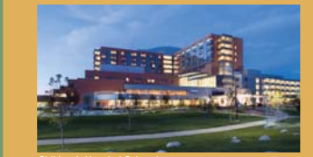
Children's Hospital Colorado Aurora, Colorado
