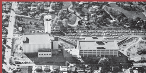
Mountain Bell Zuni Communications Center Denver, Colorado
